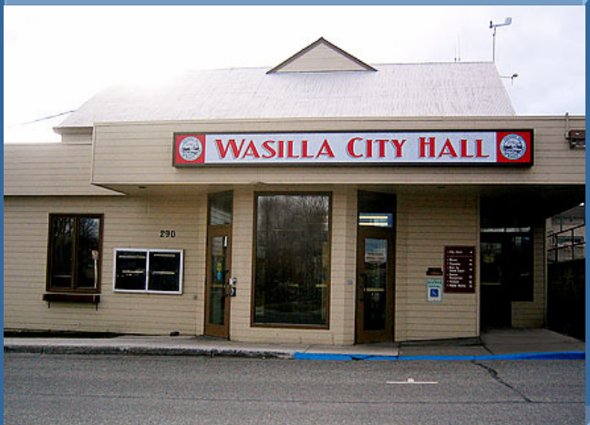
Wasilla's City Hall, where Palin was once employed. Note how it looks like a store in a strip mall. IMAGE COURTESY: AKMuckraker (akmuckraker@yahoo.com)
